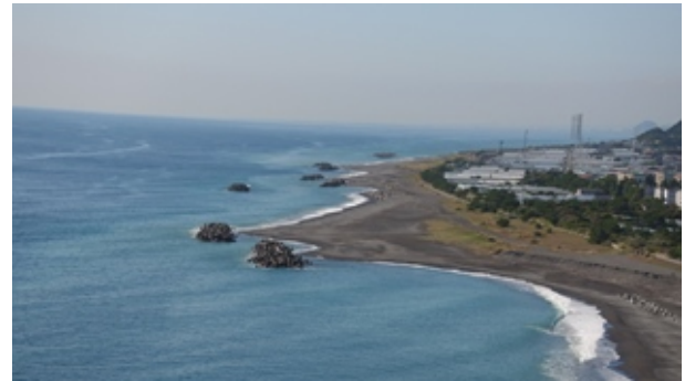
Fig.1 Coastal shore erosion and wave dissipating blocks
