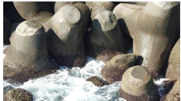
Fig.10 Downward sagging area of the blocks
