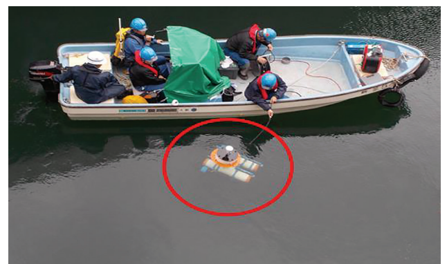
Figure 9 | Approach to dam with ROV.
